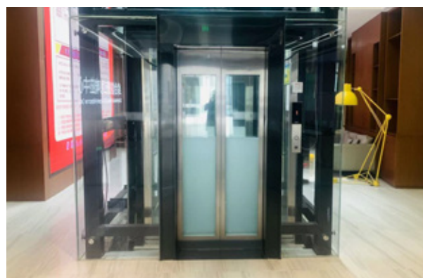
The elevator outside the Command Center
